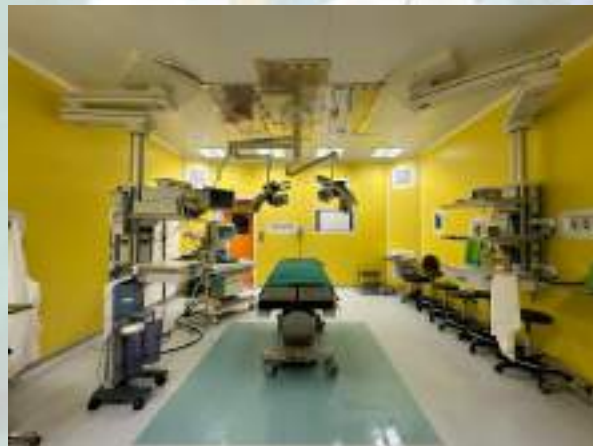
Kamar Operasi Minor Lantai Ground
